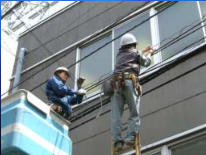
3. Running along with feeder cable
