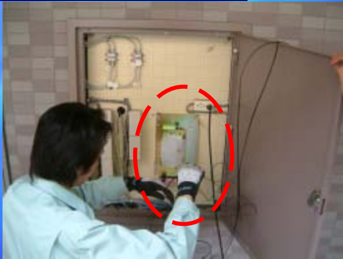
5. Connected to a 1x8 splitter within the MDF
