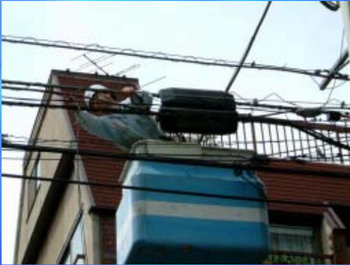
1. Installation of closure
