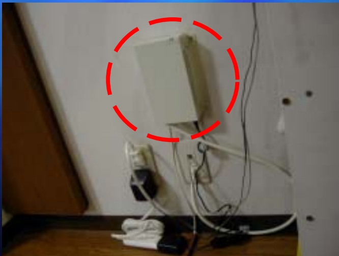
11. ONU is fixed on to the wall
