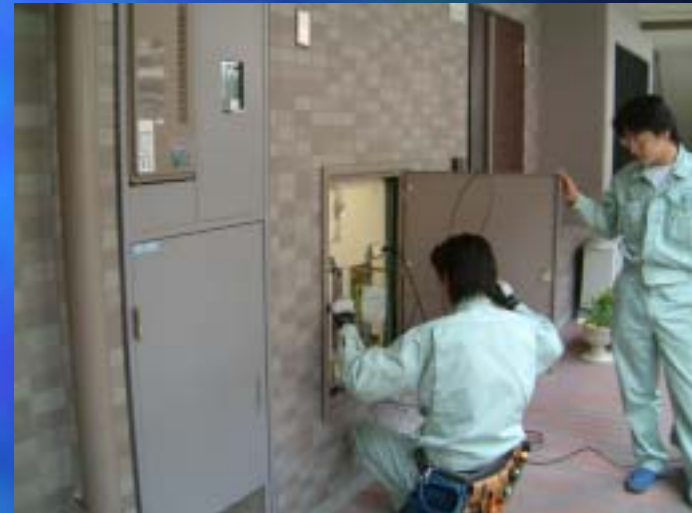
6. Cable pulled through vertical conduit from MDF to IDF
