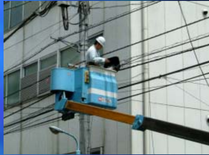
2. Splicing within closure
